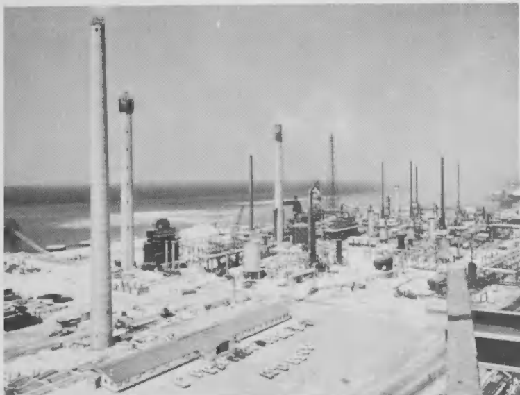
HDS Facilities, Phase II, under construction. Facilidad HDS-II bao construccion.
